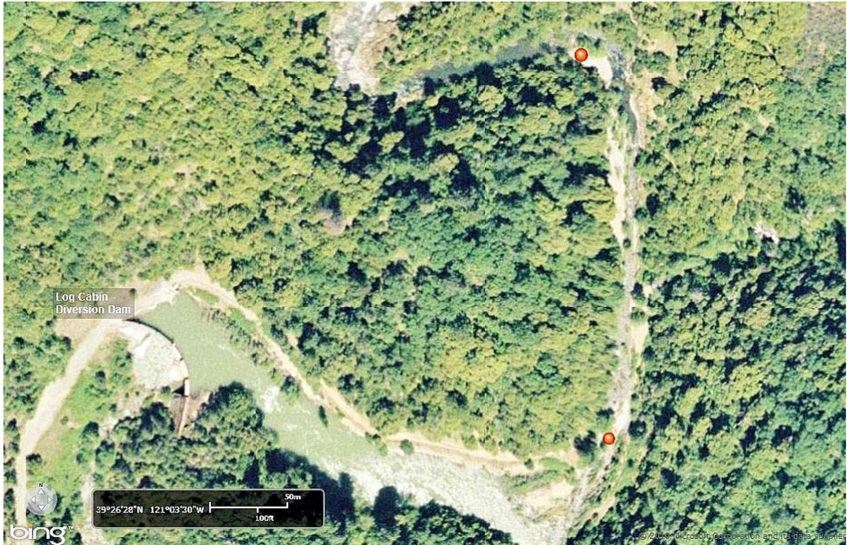
Figure 5.0-4. Oregon Creek Non-Project Affected Reach: aerial image of downstream section investigated in March 2011. The approximate extent of the March 2011 reconnaissance area is demarcated by red dots.
